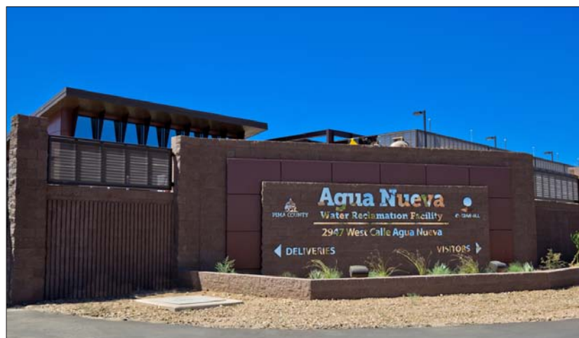
Agua Nueva Water Reclamation Facility / Built through a P3 process by Pima County and private partners
